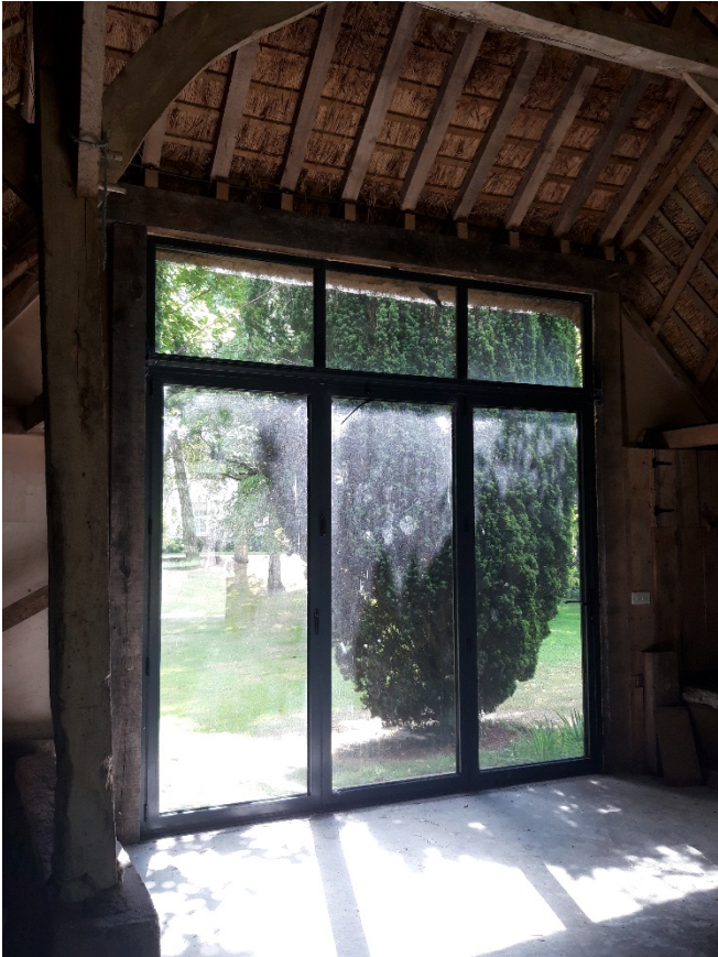
Internal view of South elevation, August 2020
